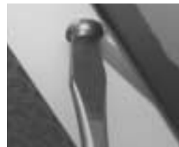
Stainless screws draw door frame tight. Fasteners are captive and frame is supported by chains.
