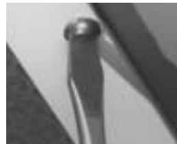
Stainless steel screws draw door frame tight. Fasteners are captive and frame is supported by chains.
